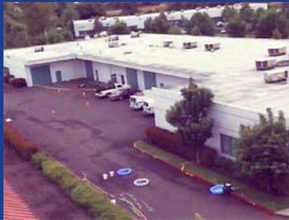
The H2O Technologies plant in Milwaukie. (KGW Photo)
