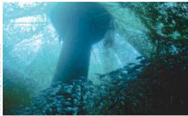
Fish-eye view—Hawai'i Sea Grant researchers successfully used giant sea cages to grow thousands of moi, favored fish of traditional Hawaiian fishpond aquaculture. The 50-by-80-foot conical sea cage is made of steel and NASA-developed mesh designed to withstand 25-foot waves. It was moored 40 feet below the surface two miles off the 'Ewa O'ahu shore. Researchers predict open-ocean mariculture could become a $100-million-a-year industry.
