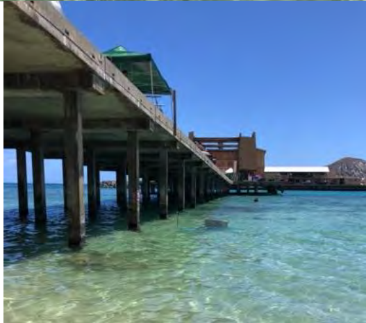
Figure 2. Flap testing at the Makai Research Pier.
