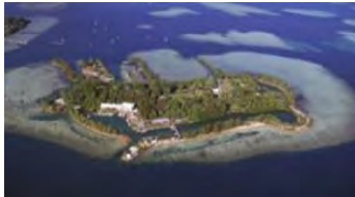
Figure 1. DC microgrid project site, Coconut Island.
