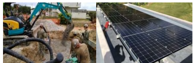
Figure 3. Project construction and new PV system.
