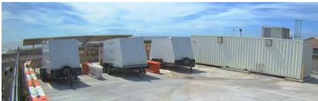
Figure 5. Hydrogen Transport Trailers.
