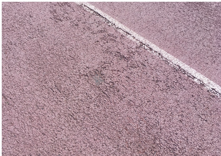
Close up of deteriorated track surface
