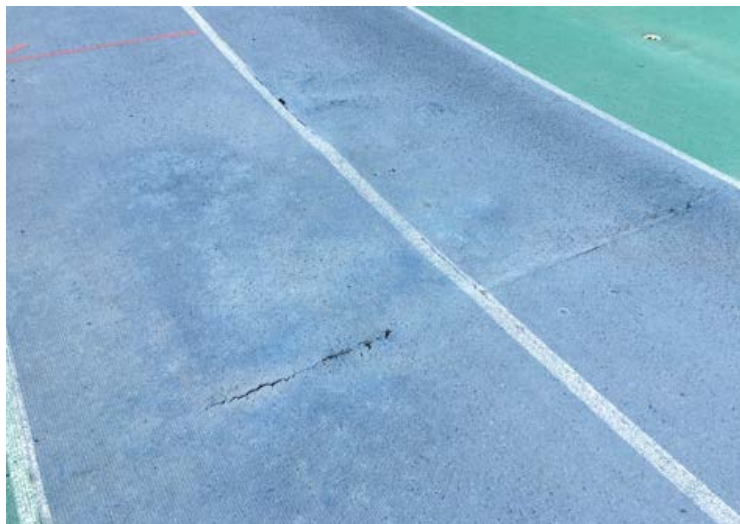
Cracks in track surface
