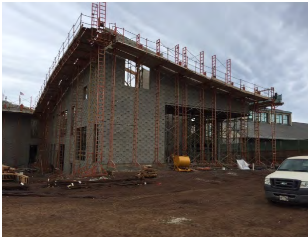
Entrance to administration wing – north side
