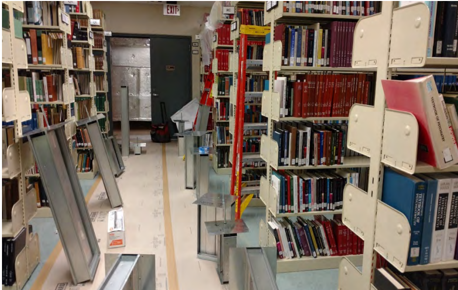
Install motorized dampers
