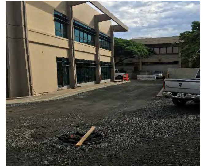
South side of the building – subbase being installed prior to asphalt concrete pavement
