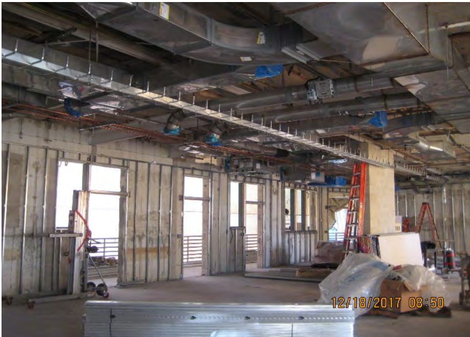
Ceiling coordination and installation; mechanical, electrical, plumbing and communication trays
