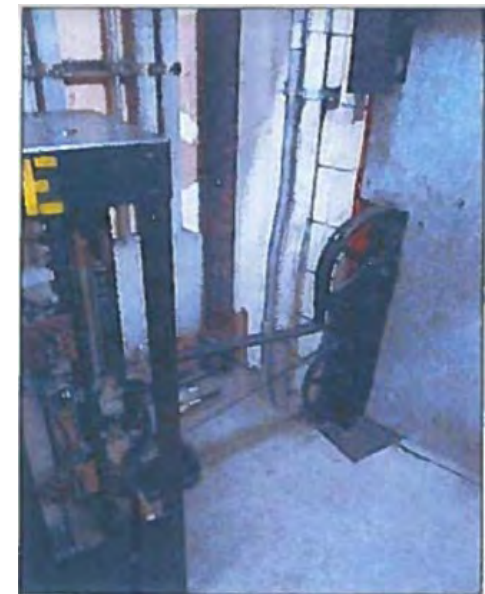
Shidler elevator machine room that will be modernized
