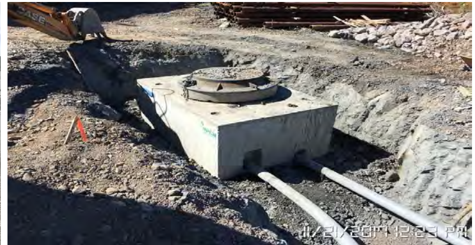
New Hawaiian Telecom manhole and conduit installed at Lilipuna pier
