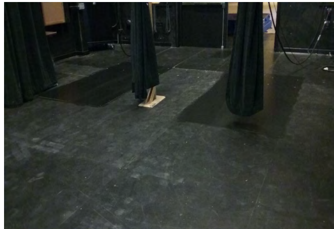
Ernst Lab Theater Makai-side floor repairs painted black
