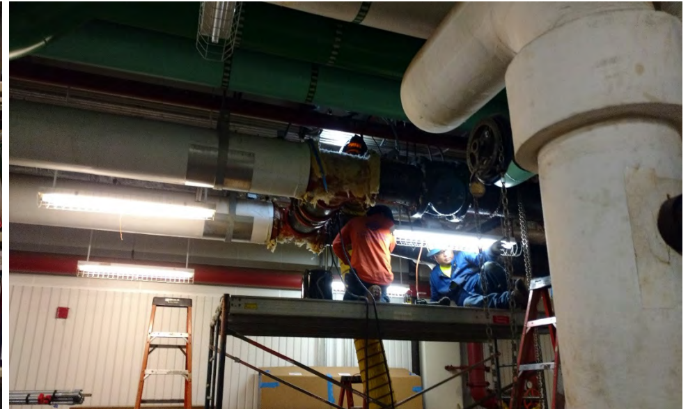
Weld supports for chilled waterline
