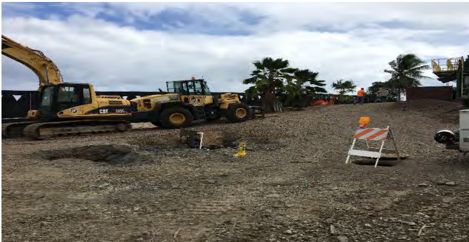
Excavation for new waterline at Lilipuna Pier
