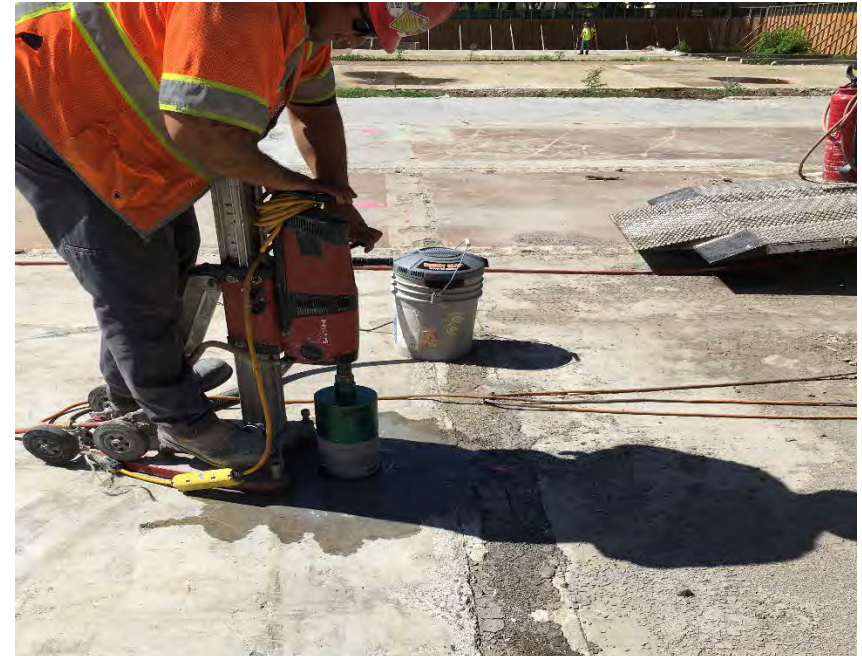
Soil testing to determine the extent of the hazardous conditions
