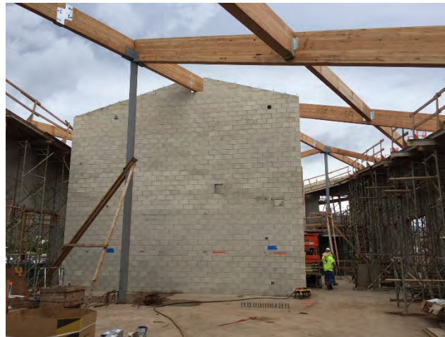
Administration wing – second floor open office area
