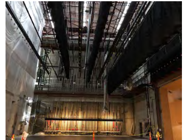
Rigging system, stage curtains and lighting, catwalk, stage and lift flooring/coating
