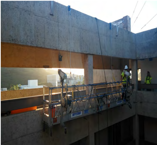
Atrium spall demo
