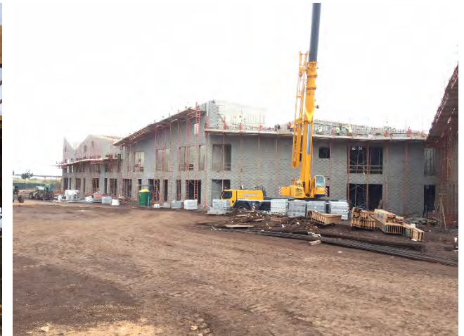
Classroom wing – north side
