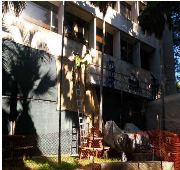
Spall demo on South East side of building
