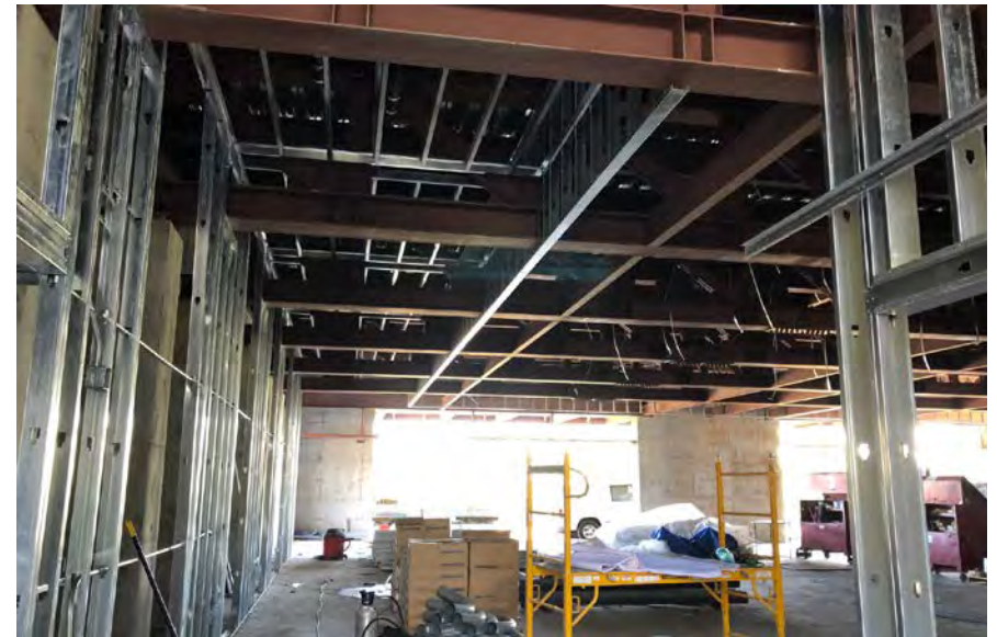
Metal framing on Level 1
