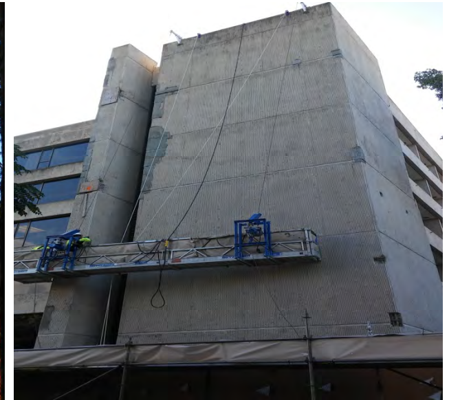
Spall patching on North side of building
