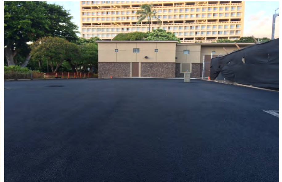
Completed asphalt concrete pavement
