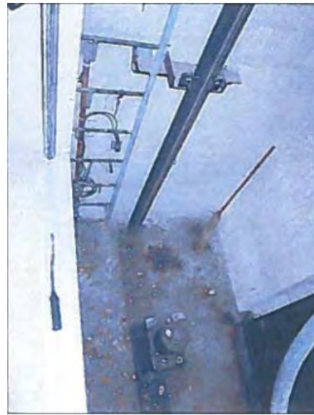
Shidler elevator pit
