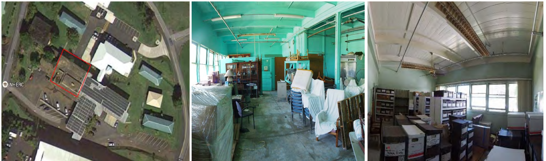
Existing unused wing at NHERC which will be renovated
