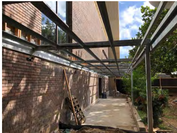
Exterior canopies, wall restoration and side entries
