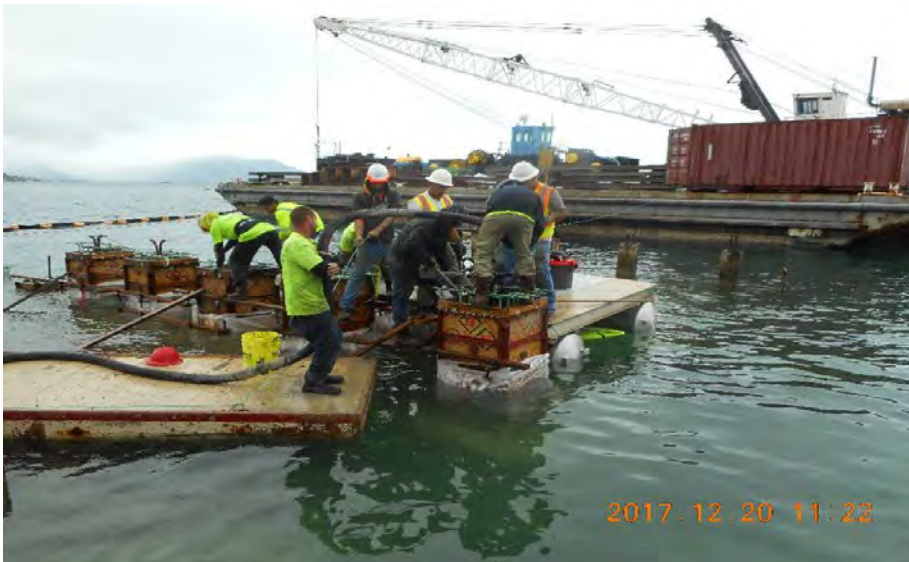
Concrete tremie pour at bent 15, at the end of the pier with new deck planks
