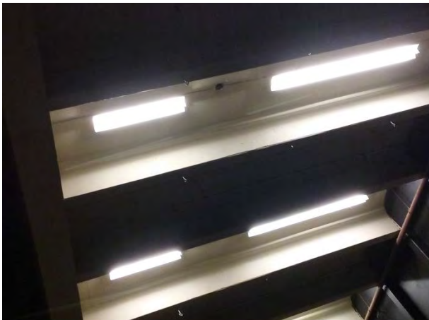
Completed installation of Upper Main Stage high bay light fixtures
