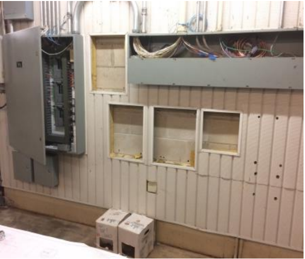
Removal and installation of new control boxes
