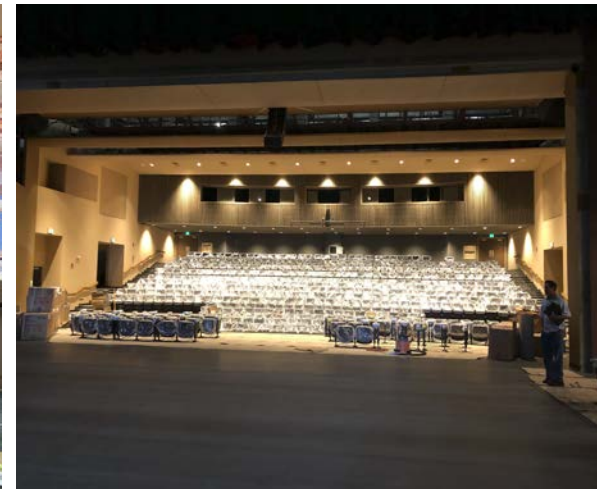
Work on auditorium seating, flooring, lighting, painting, audio, etc. ongoing
