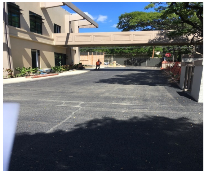
Asphalt pavement completed
