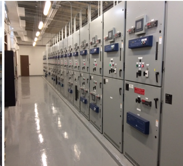
Substation M – Switchgear Room
