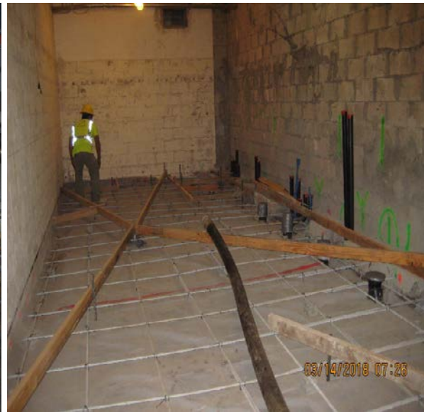
Underground plumbing of sanitary waste lines and venting in restroom; concrete forms, reinforcement and vapor barrier in place
