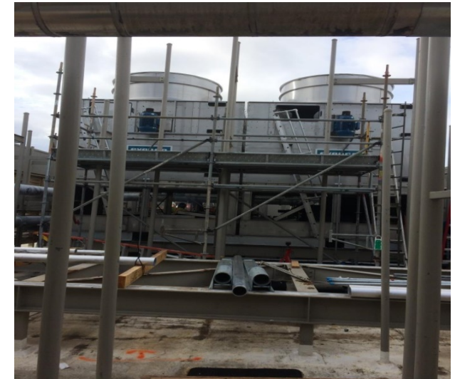
Weld supports for new cooling towers
