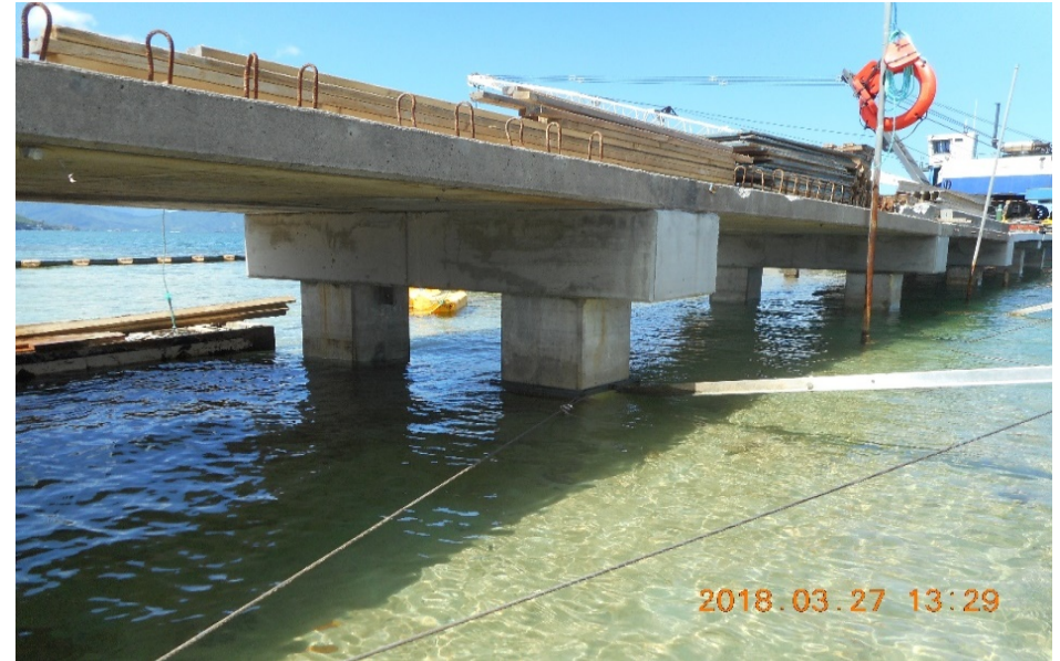
New concrete encasement of pile caps at underside of existing decking completed
