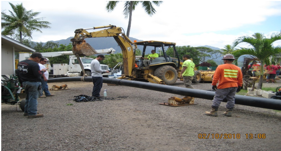
Installation of the new waterline
