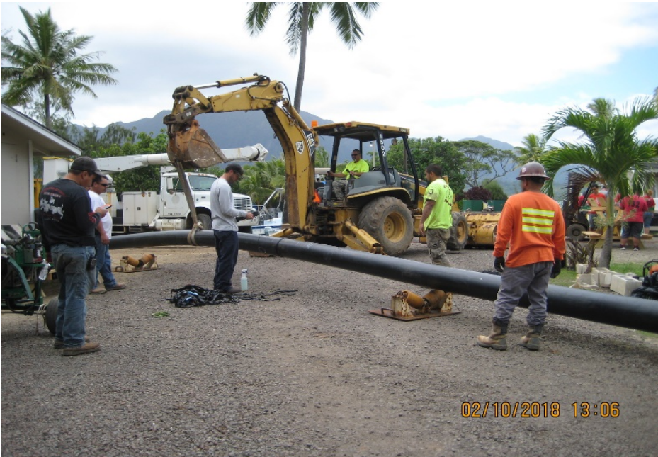
Installation of the new waterline
