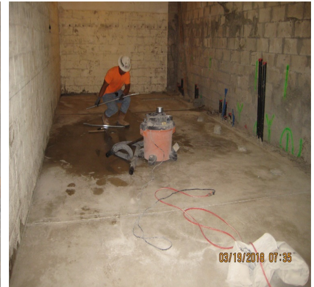
Concrete placed at restrooms with control joints being placed to locate cracking at resinous floor joints
