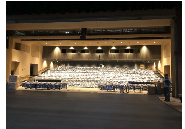
Work on auditorium seating, flooring, lighting, painting, audio, etc. ongoing
