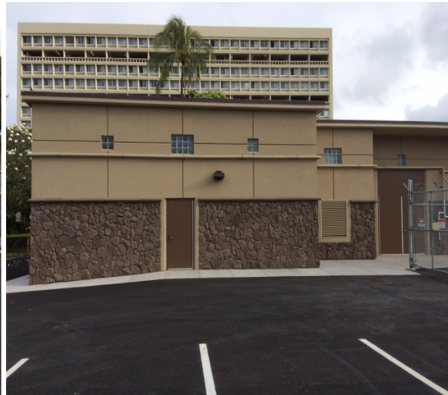
Completed Substation M (Hale Mānoa in background)
