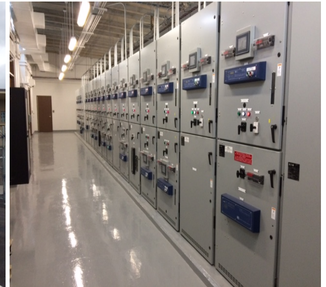
Substation M – Switchgear Room
