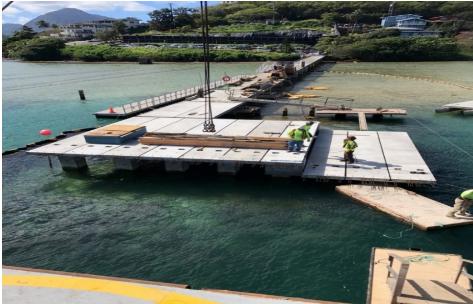
Deck planks installed over new concrete enforced piles and pile caps from bent 14 to the end of the pier with new deck planks
