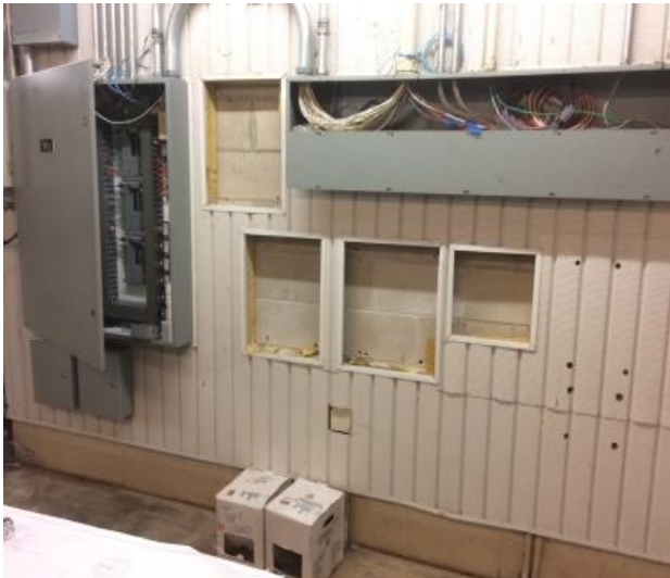
Removal and installation of new control boxes
