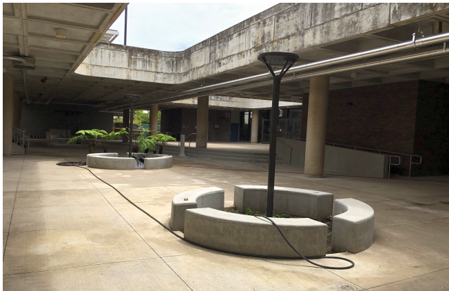
Exterior waiting area, Ticket Office, Concession Booth, Restrooms and entry to the Main Lobby
