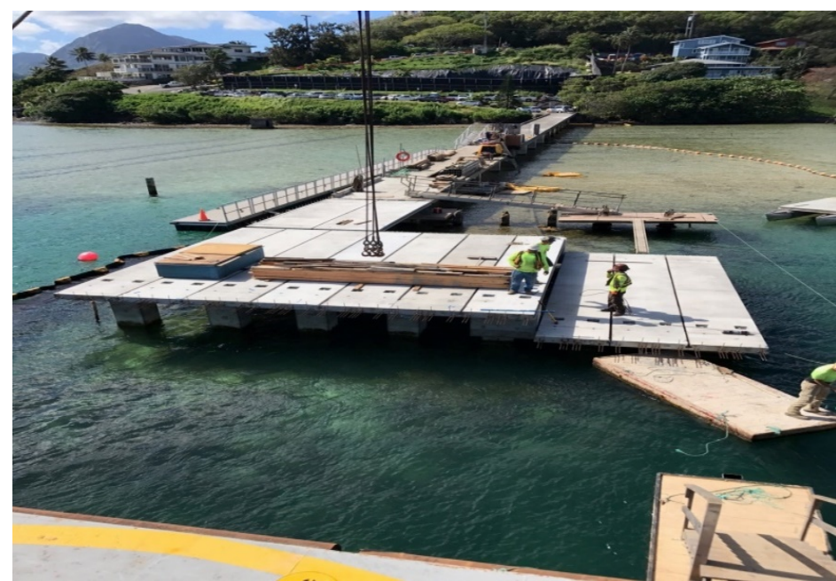
Deck planks installed over new concrete enforced piles and pile caps from bent 14 to the end of the pier with new deck planks
