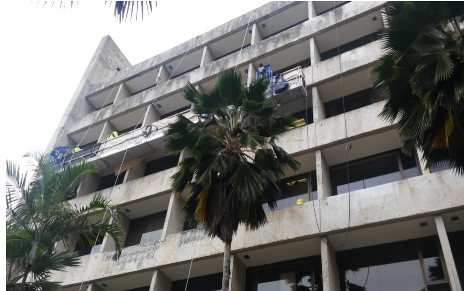
Spall and crack repair on South East Elevation drop #2
