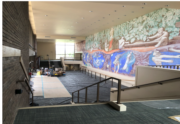
Work on Main Lobby/Entry interior ongoing
