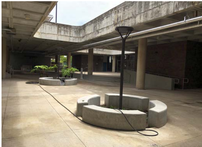
Exterior waiting area, ticket office, concession booth, restrooms and entry to the main lobby
