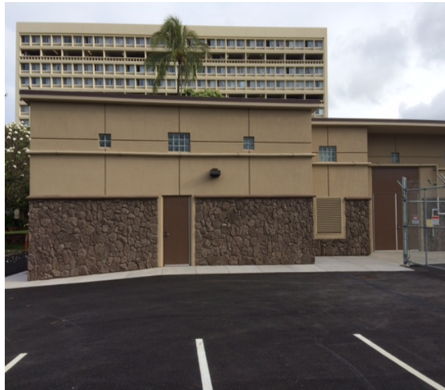
Completed Substation M (Hale Mānoa in background)
