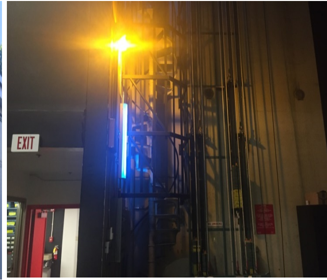
Completed safety cage around existing spiral staircase
