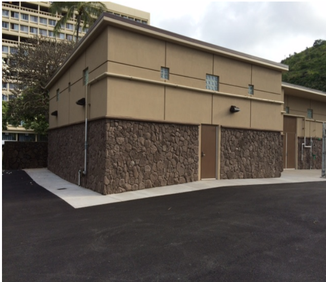
Completed Substation M
