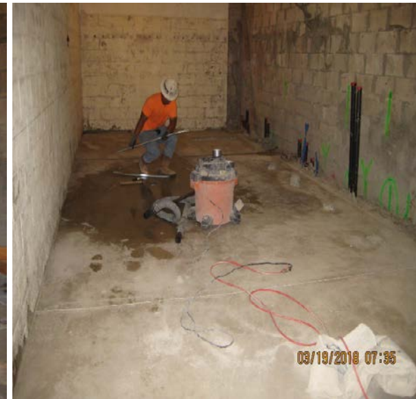
Concrete placed at restrooms with control joints being placed to locate cracking at resinous floor joints
