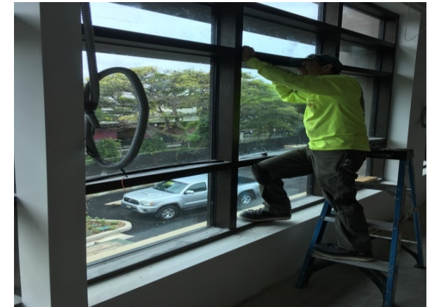
Installation of windows on second floor
