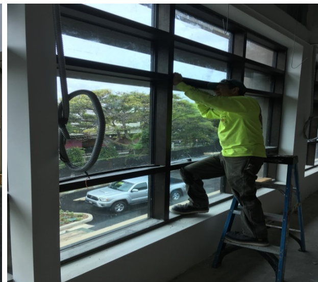
Installation of windows on second floor
