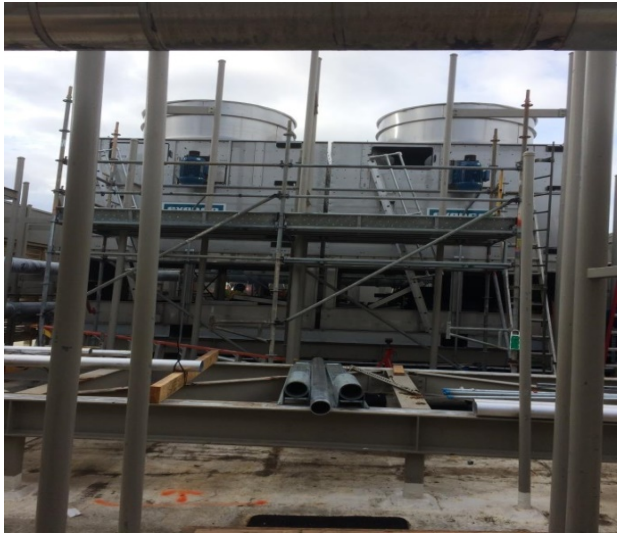
Weld supports for new cooling towers
