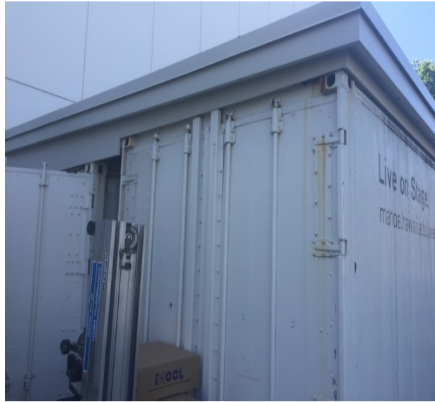
Completed roof repairs to the outside storage containers
