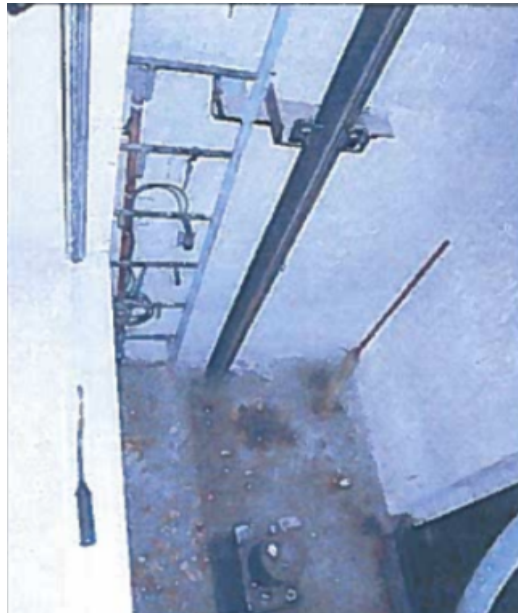
Shidler elevator pit
