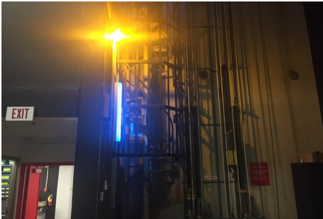
Completed safety cage around existing spiral staircase
