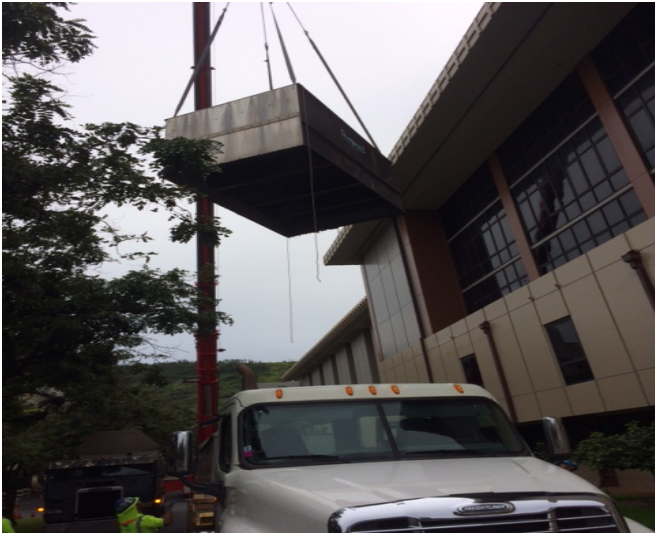
Removal of existing cooling towers
