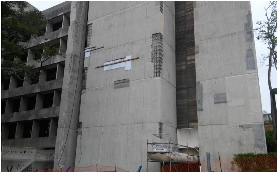
Spall and crack repair on East Elevation drop #4
