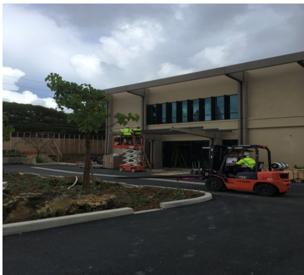
Installation of polycarbonate canopy (AC pavement and landscaping complete)
