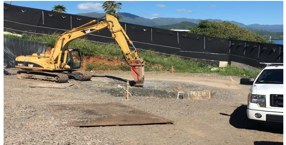
Contractor trenching to tie in the new waterline to the Board of Water Supply
