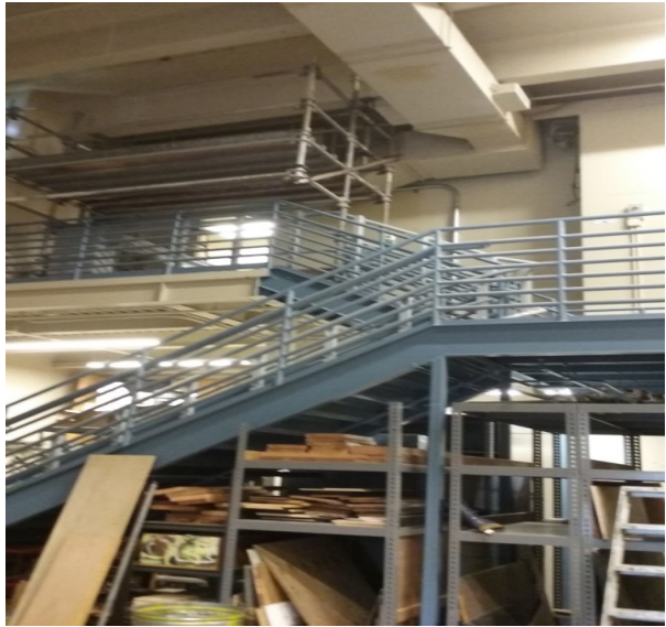
Scene shop stairs to new upstairs office
