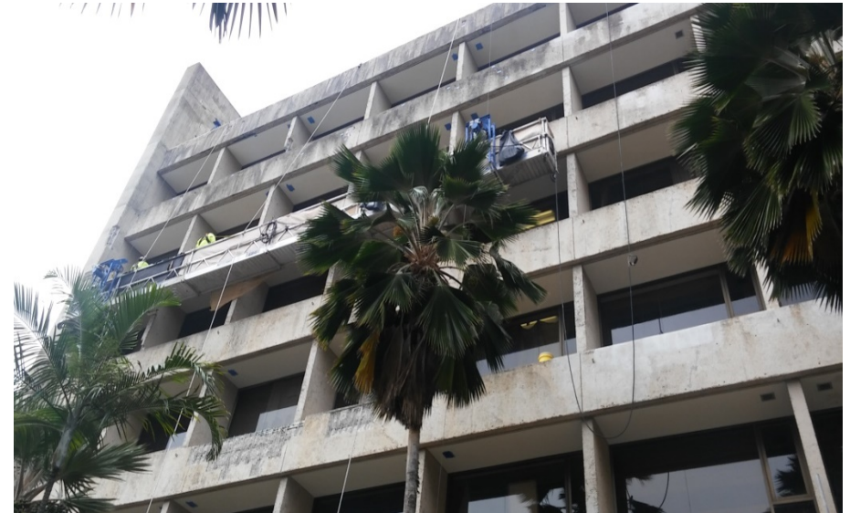
Spall and crack repair on South East Elevation drop #2
