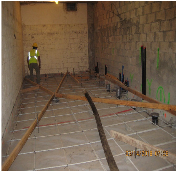
Underground plumbing of sanitary waste lines and venting at women’s restroom completed. Concrete forms, reinforcement and vapor barrier in place; ready for concrete
