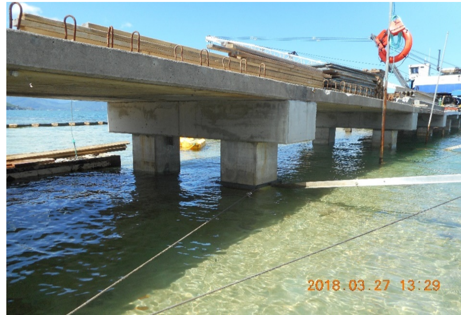
New concrete encasement of pile caps at underside of existing decking completed
