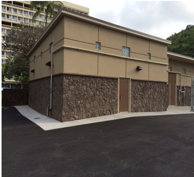
Completed Substation M
