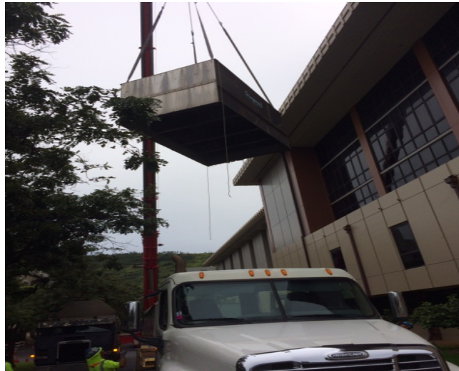
Removal of existing cooling towers
