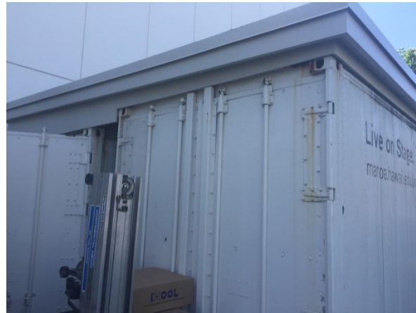
Completed roof repairs to the outside storage containers
