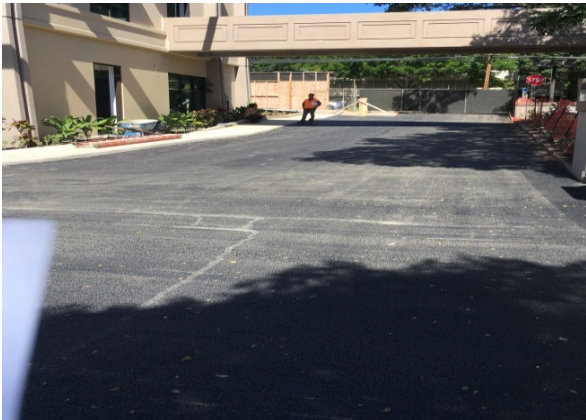
Asphalt pavement completed
