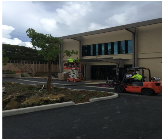
Installation of polycarbonate canopy (AC pavement and landscaping complete)
