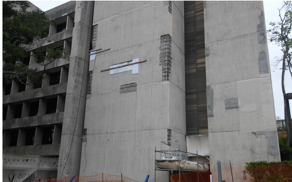
Spall and crack repair on East Elevation drop #4
