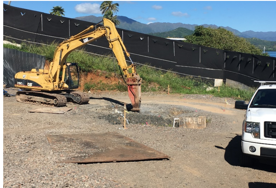
Contractor trenching to tie in the new waterline to the Board of Water Supply
