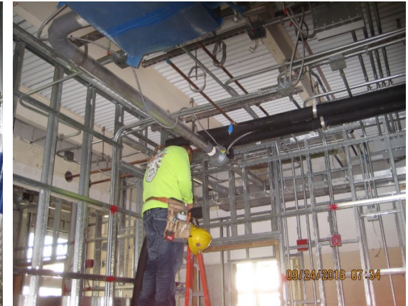
Adjustments being made to the air conditioning system fresh air intake fans
