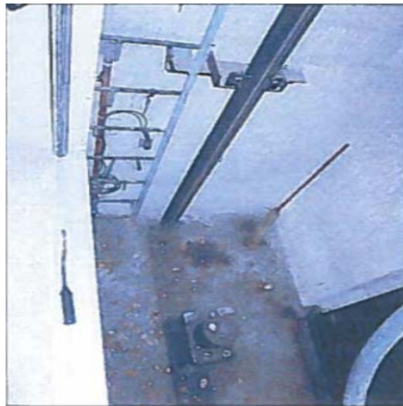
Shidler elevator pit
