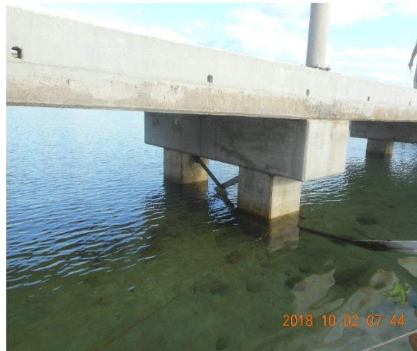
Moment-resisting structural framing at Bent 12
