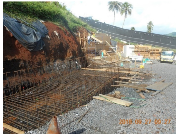
Steel reinforcement installed for the next section of the footing pour
