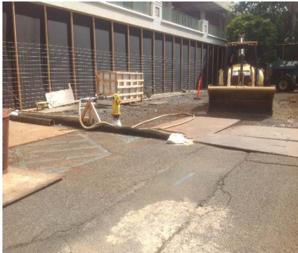
Excavation work and new fire hydrant installation
