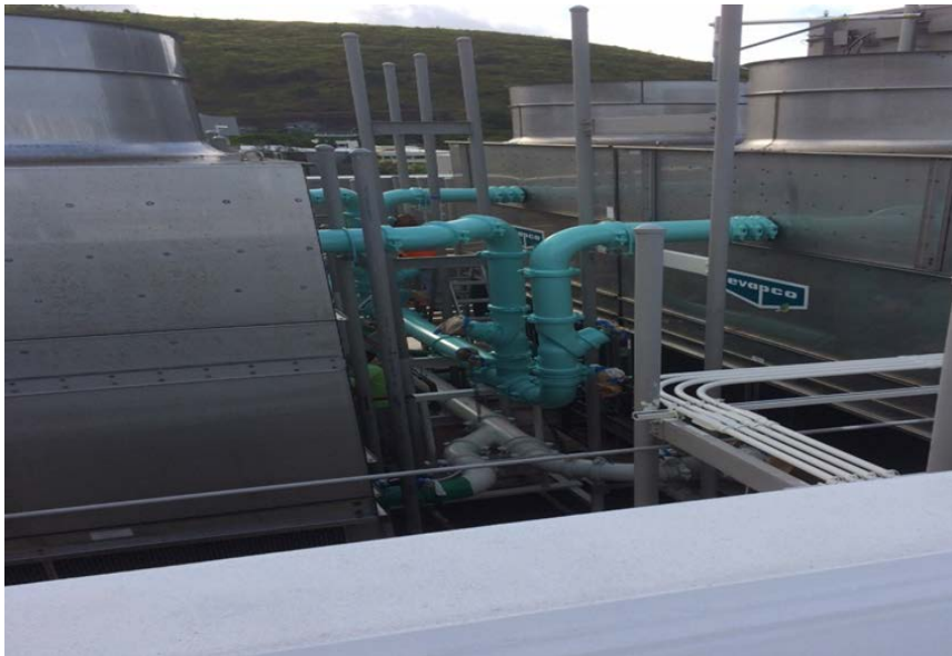
Painted pipe fittings
