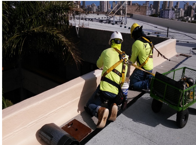
Application of fluid-applied coating on upper roof parapet walls
