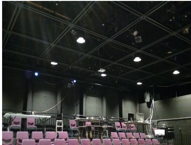
Ernst Lab Theater tensioned wire grid
