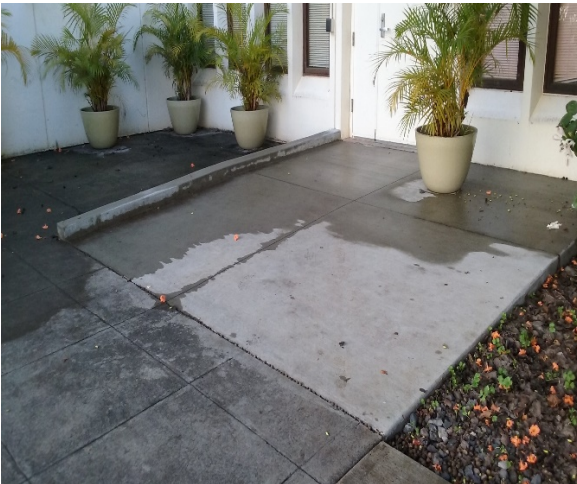
Ewa entry ramp
