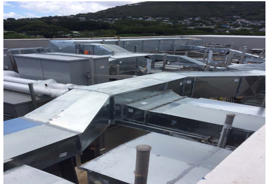
Sheet metal roofs installed over exterior ducts
