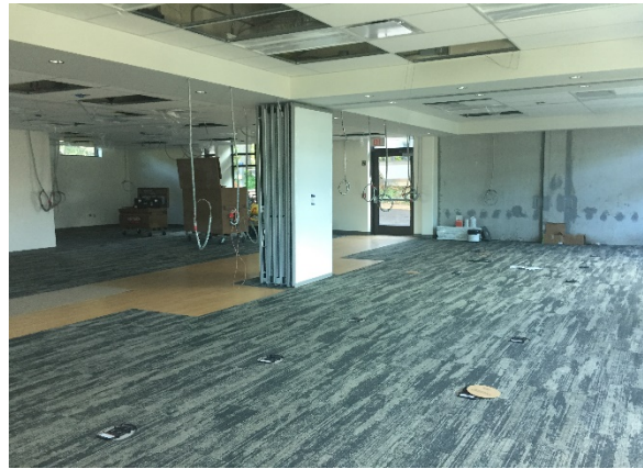
First floor interior – future classroom space
