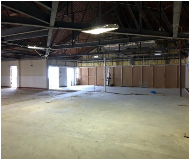
East-Facing 2nd Floor: Demolition complete; laying out new walls and rough-ins
