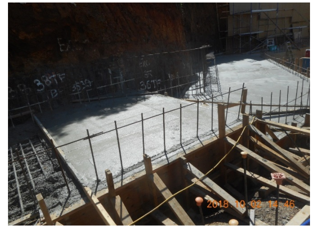
Footing for the next section of the wall
