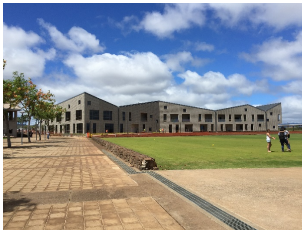
Exterior view from southwest
