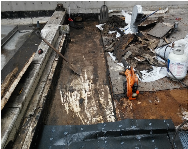
Demolition of Saunders Mechanical Building roof
