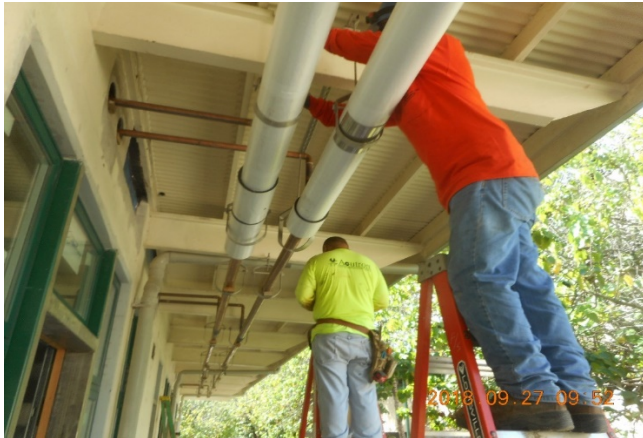
Chilled water lines being insulated
