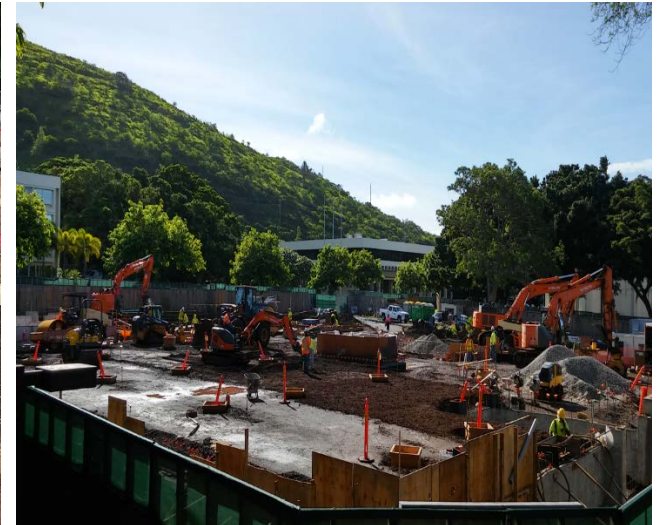
Grading and foundation work (viewed from northwest corner of site)
