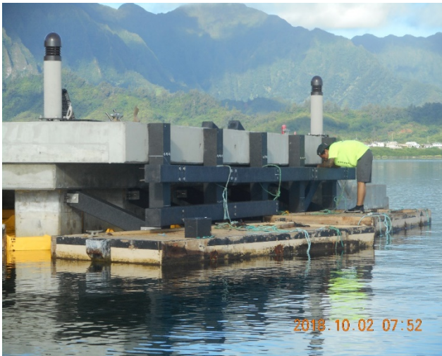
Ongoing front fender installation
