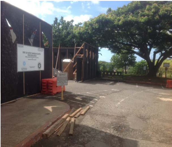
Barricade and staging area entry
