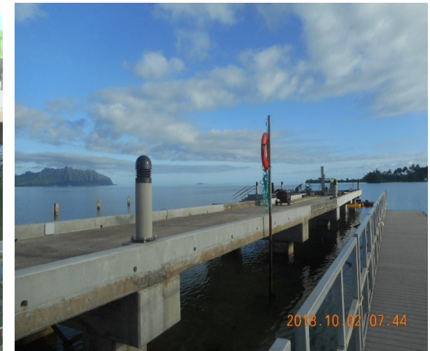
Concrete curbs with new bollard light fixtures
