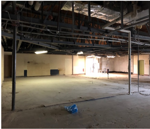
West-Facing 2nd Floor: Demolition complete; laying out new walls and rough-ins
