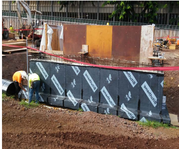
Elevator pit walls and waterproofing
