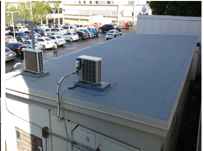
New roof over costume containers
