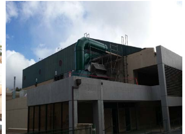
Gym 2 new air conditioning equipment
