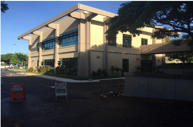
East facing side of the building – site work complete and inspected and punch list provided
