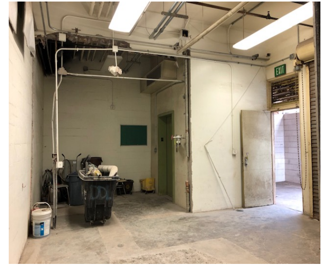
1st Floor Loading Area: Demolition of walls and utilities; prepping new layout
