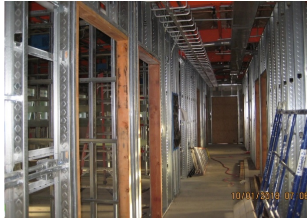
Drywall framing completed in the upper floors
