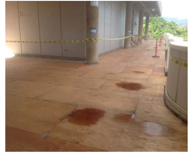
Second floor exterior deck demolition work
