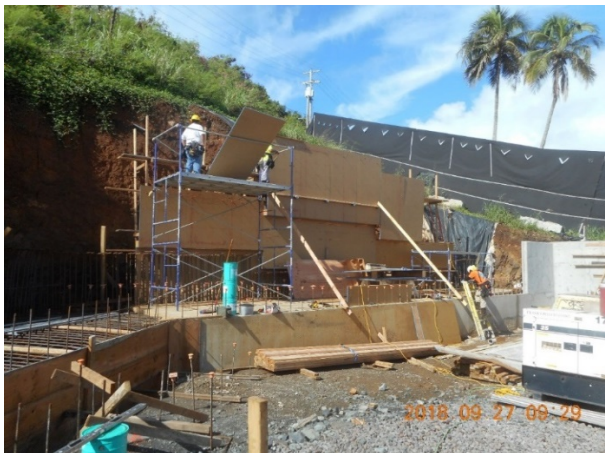
Half of the concrete footing for the retaining wall completed; forms being installed for the higher wall.
