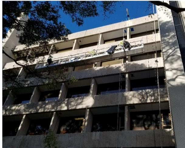
*Fluid Applied Coating on East Elevation Ledges*
