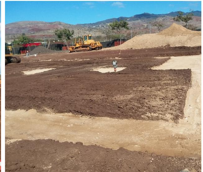
*Excavation of Building Wall Footings and Compaction of Select Coral Fill Material*
