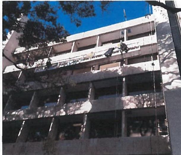
***Fluid Applied Coating on East Elevation Ledges***
