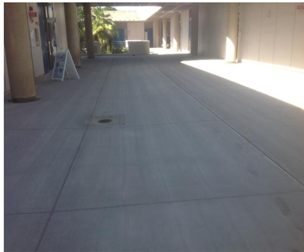
*Preparation of the 2nd floor - new exterior deck infill, drains and expansion joint for the application of the new deck coating system*
