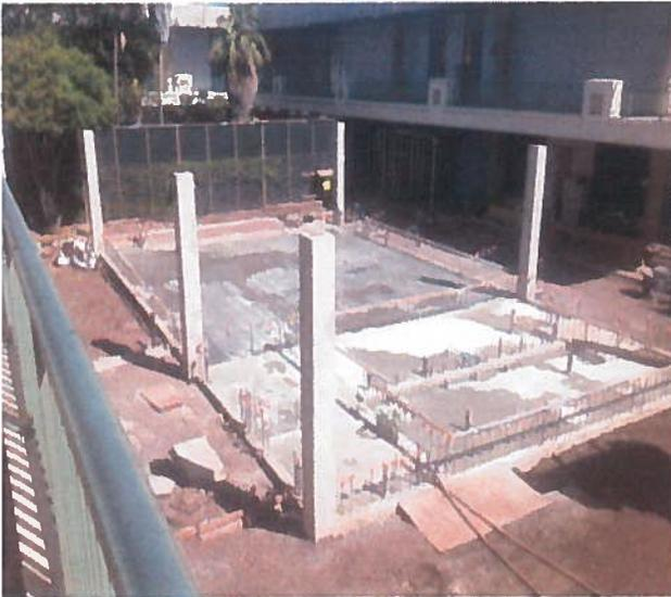
***Erection of the structural columns, plumbing piping and rough-ins for the new Dance Studio addition***
