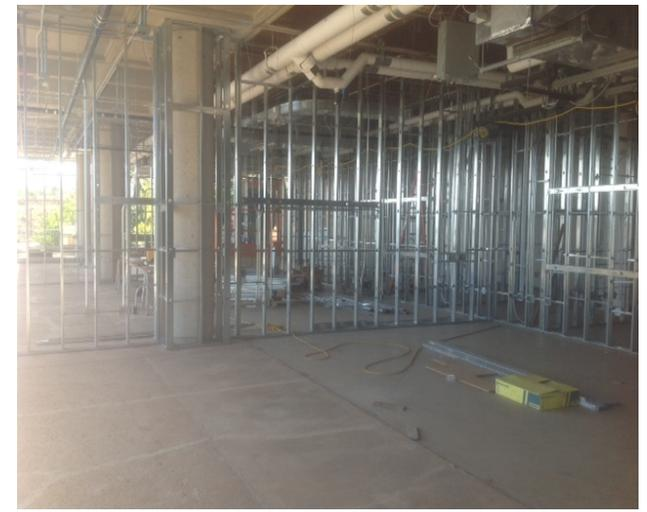
*Ground floor interior utilities rough-ins and stud wall framing*
