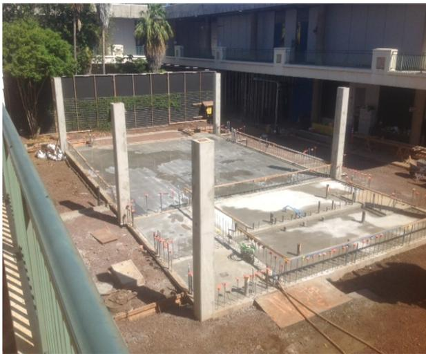
*Erection of the structural columns, plumbing piping and rough-ins for the new Dance Studio addition*
