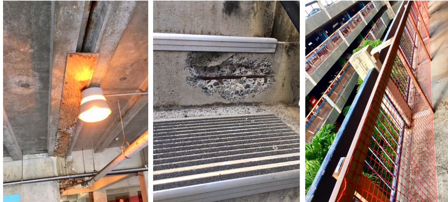
Current Condition of Parking Structure Phase I
