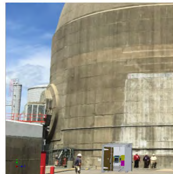
Potential deployment with shield (above left) at North Anna reactor (above)
