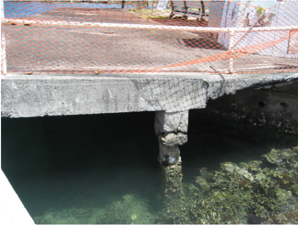
Pier support columns are eroded and unsafe
