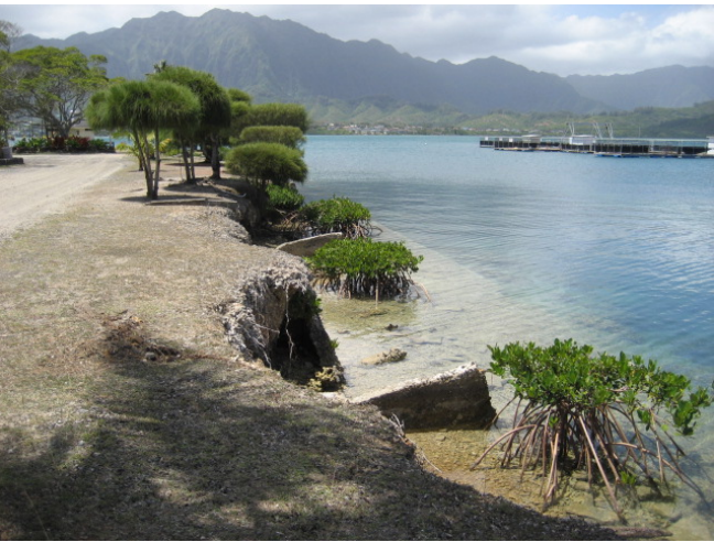
Eroding seawall inner channel
