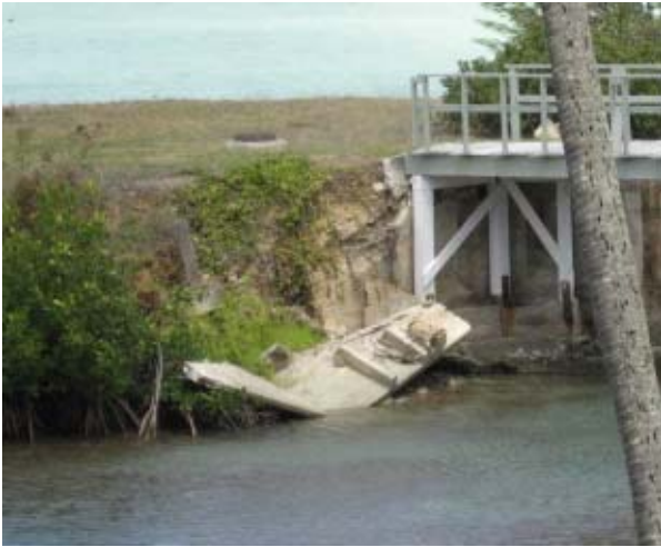
Fallen seawall, inner lagoon
