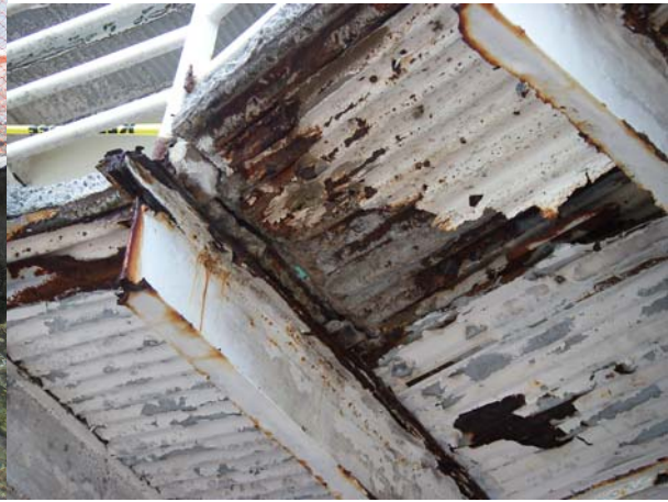
Pier support columns are eroded,unsafe Walkways on buildings are rusting, unsafe.
