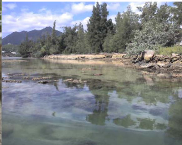
Eroding seawall inner channel
