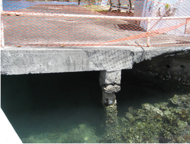
Pier support columns are eroded,unsafe Walkways on buildings are rusting, unsafe.
