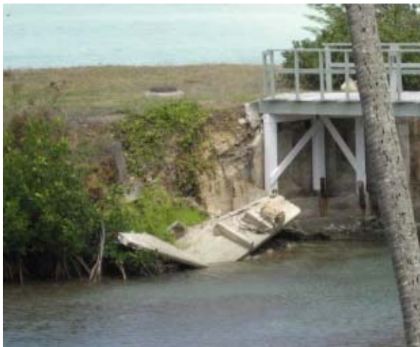
Fallen seawall, inner lagoon
