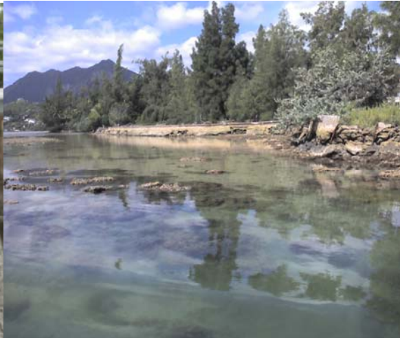
Eroding seawall inner channel
