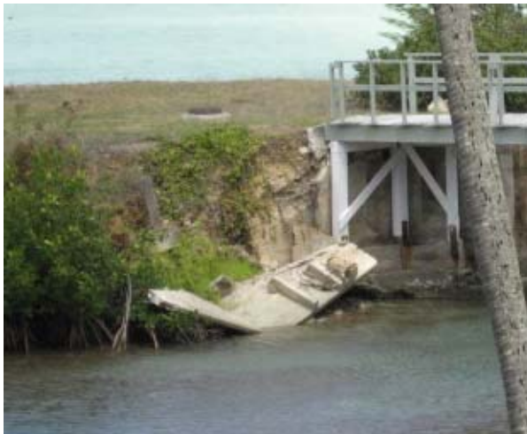
Fallen seawall, inner lagoon
