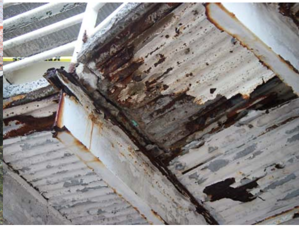
Walkways on buildings are rusting, unsafe.
