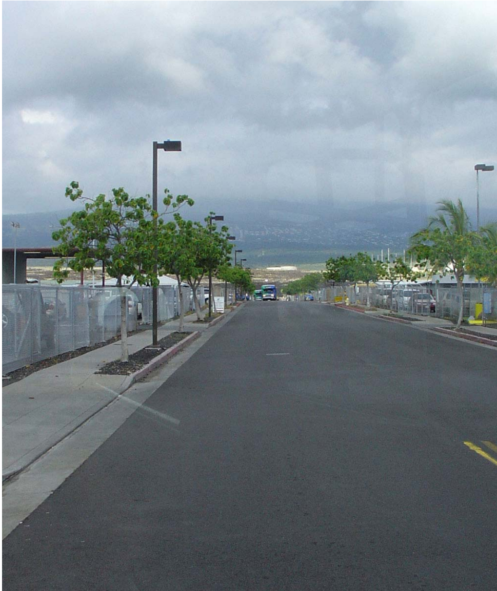
Newly installed lighting on the roadway at Kona airport near the car rental lots. These lights are high-pressure sodium. The Hawaii county lighting ordinance requires use of low-pressure sodium lamps for roadways.
