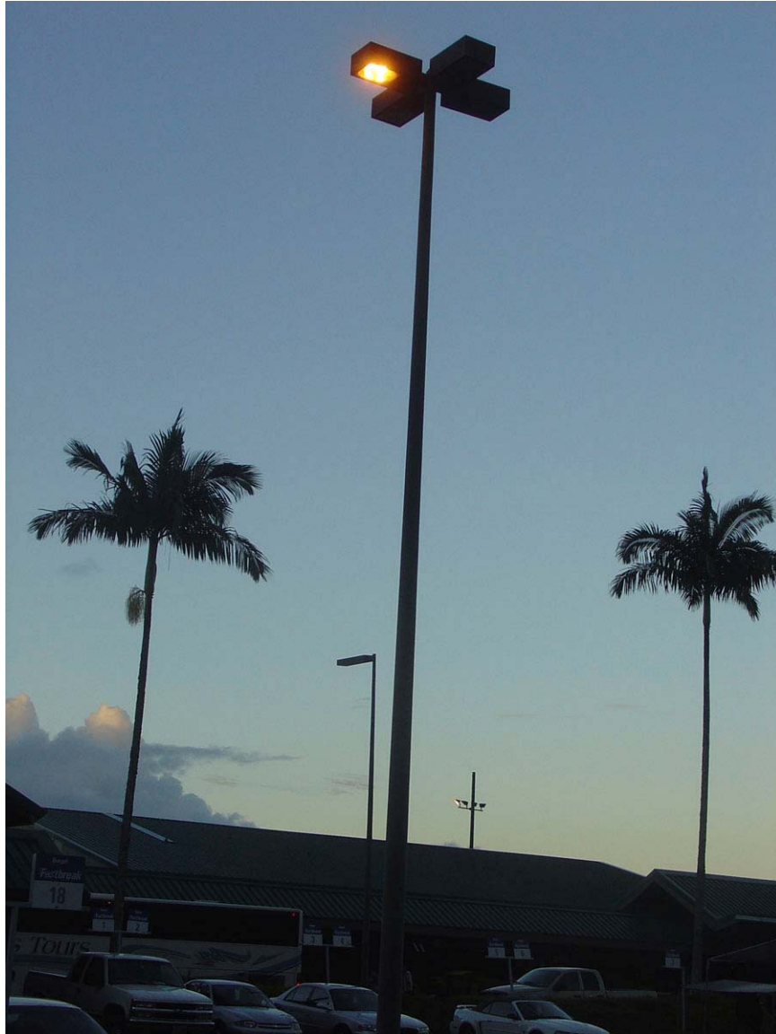
Newly installed parking lot lighting in Hilo airport. These lights are high-pressure sodium lamps. The Hawaii county ordinance requires parking lots to be lit using low-pressure sodium lamps.
