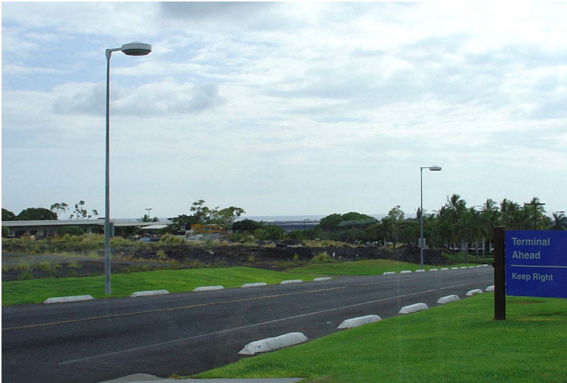
High-pressure sodium lamps along the access road to the Kona airport. The Hawaii county lighting ordinance requires use of low-pressure sodium lamps on roadways.
