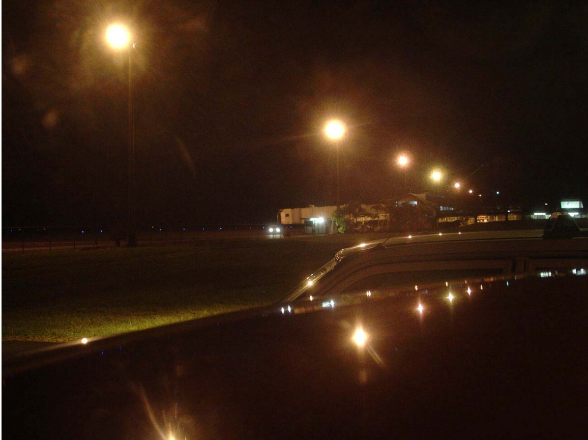
Ramp lighting at Hilo airport. These lights should be fully shielded to conform to the Hawaii county ordinance. They are not properly shielded.
