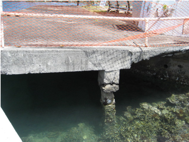
Pier support columns are eroded and unsafe
