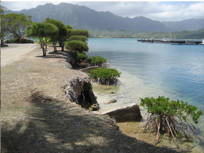
Eroding seawall inner channel
