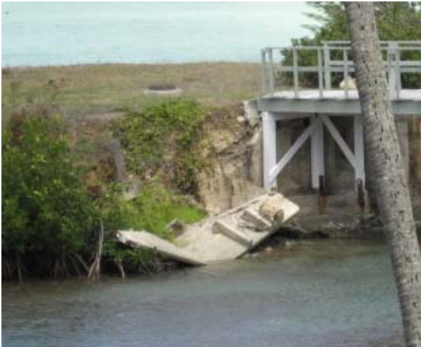
Fallen seawall, inner lagoon
